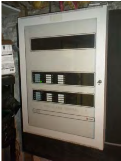
Central fire alarm control panel
