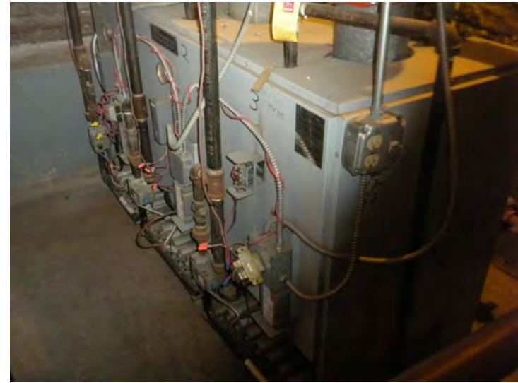
View of the central boilers – Estimated total capacity of 900 MBH
